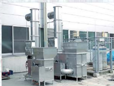
KESMAK KS-6/KS-7 Metalworking industry For hot air/oil smoke 120m 3 /min·150m 3 /min
