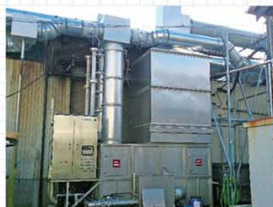
KESMAK KS600-4D Textile processing industry For odors 600m 3 /min
